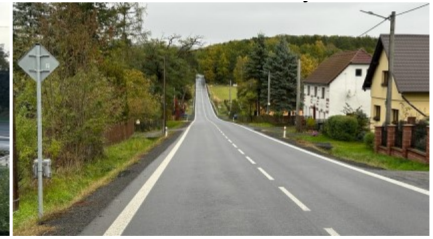
Velká Bukovina - Karlovka, 523 inhabitants, 50.7425131N, 14.3977703E, Class II road, 2 300 vehicles/day
