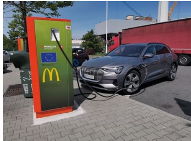
FIGURE 2. A slow-charging station in Czechia [9].
