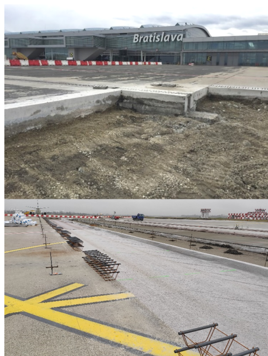
FIGURE 7. Realization of cement-concrete pavements on the Apron.
