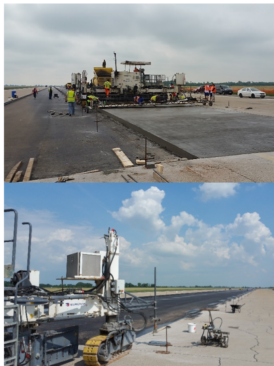
FIGURE 4. Paving of cement concrete slabs on runway 13-31.
