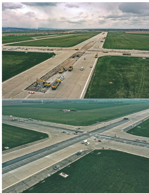
FIGURE 9. Rehabilitation of the junction of the RW 04-22 and RW 13-31.
