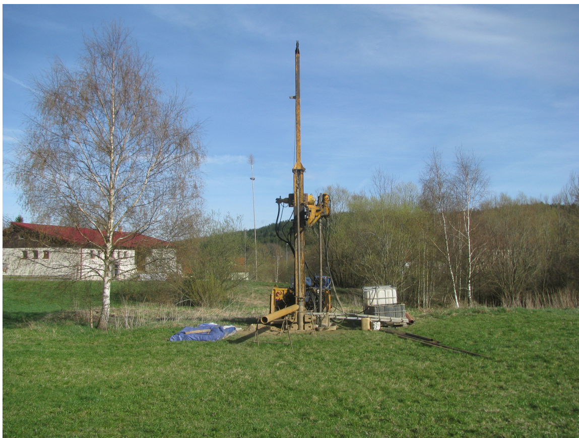
FIGURE 2. Drilling rig on site.
