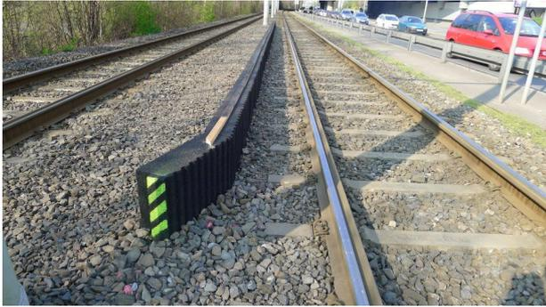
FIGURE 8. MNAS seen from the start of the section – chamfered first unit is evident in the front.
