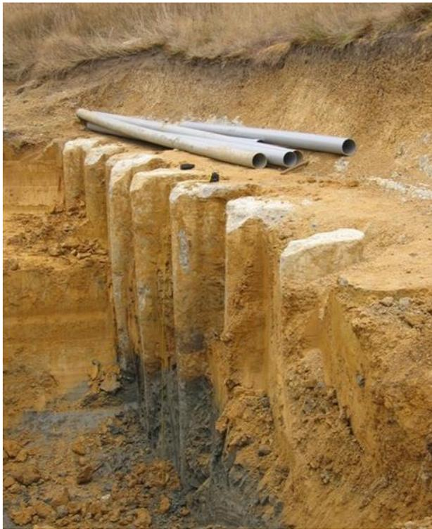
FIGURE 3. Vertical lime-cement columns – technology COLMIX [3].
