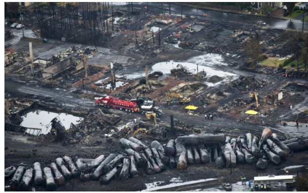
FIGURE 3. Consequences of freight train accident in Lac-Méganic, Quebec, Canada on July 6, 2013 [19].
