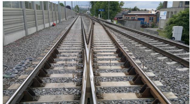
FIGURE 3. Turnout no. 4 and single crossover with turnout no. 3.
