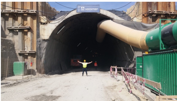
FIGURE 12. Shell structure on the western portal of the tunnel Povážský Chlmec
