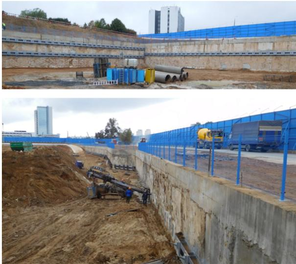
FIGURE 2. Excavation pit overview and installation of anchoring piles.
