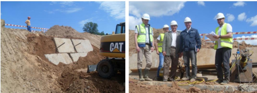
FIGURE 4. Assembling panels of support system for two experienced anchor piles and sampling testing for one of them.
