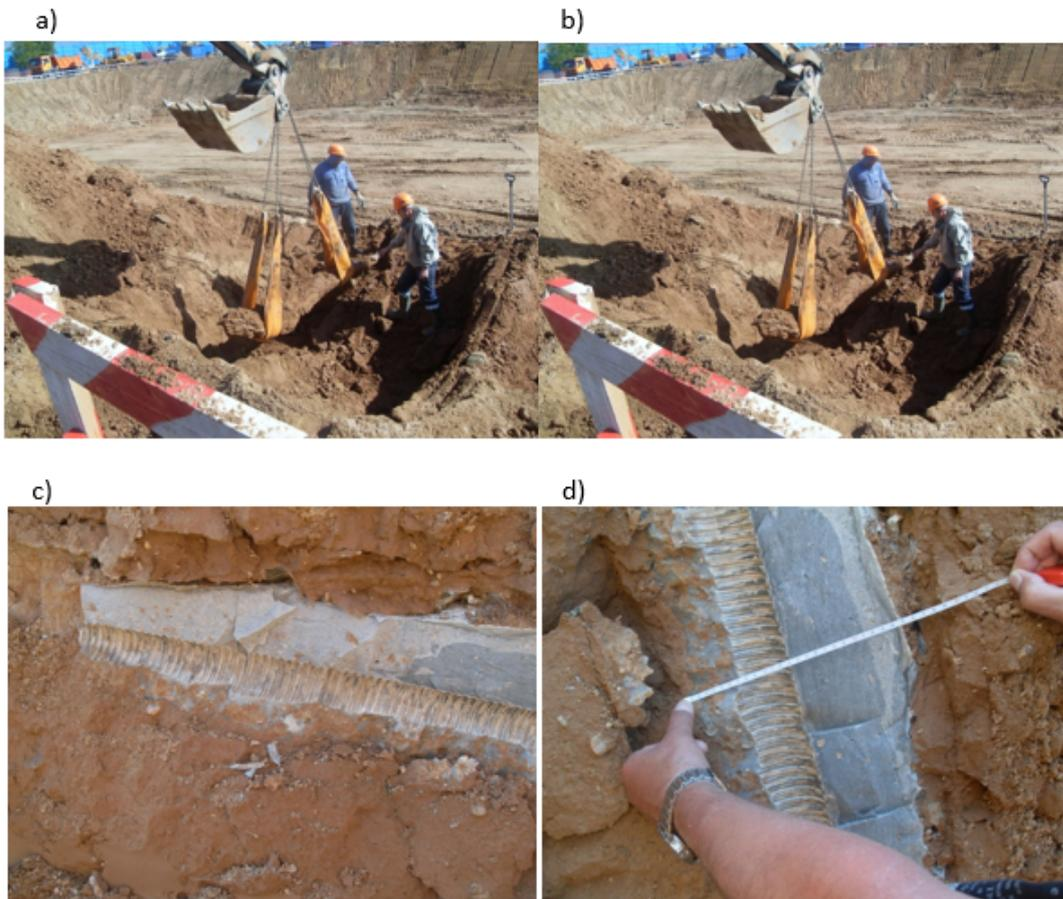
FIGURE 3. Removing from the ground (a) The form of excavated three anchor piles (b). Fragment of anchor piles body remaining in the ground (c), Measurement of the diameter on the contact with the stem (d).
