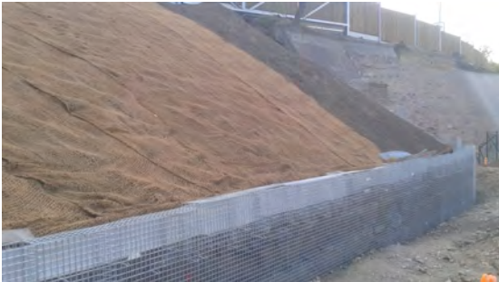
FIGURE 6. Attached front facing system MURALEX® before 63/125 mm stone filling
