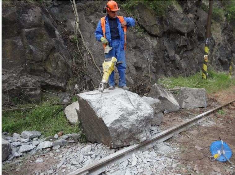
FIGURE 3. Fallen rock block after partial disintegration.
