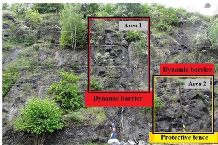
FIGURE 9. Locations for the placement of dynamic barriers and the protective fence in the endangered areas of the rock wall.
