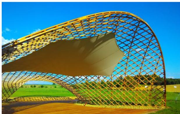
FIGURE 1. Realization of a multipurpose gridshell pavilion in Třebešov [1].
