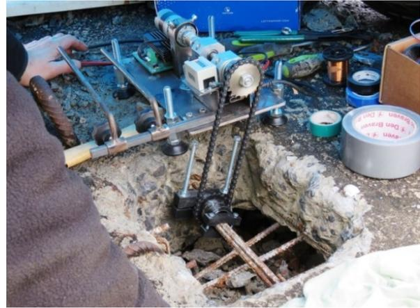
FIGURE 2. The production of the secondary coil in-situ.
