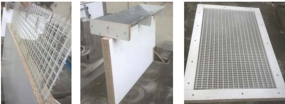
FIGURE 4. Formwork for TRLC slabs with 3D glass textile.
