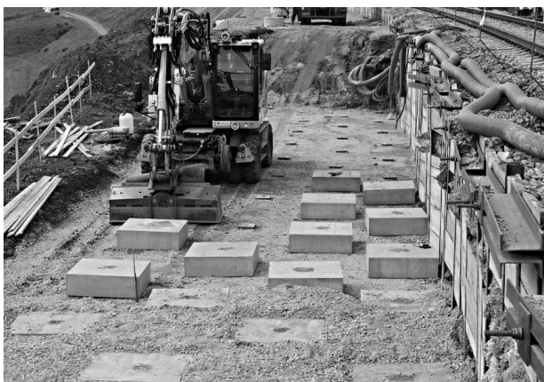
FIGURE 6. Procedure of the spreading heads under the track No. 1.
