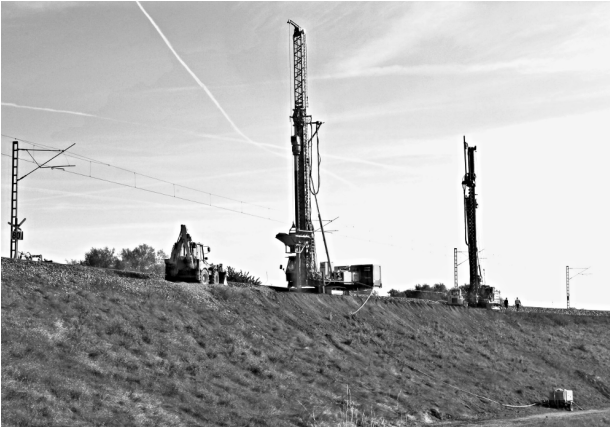
FIGURE 8. Vibro-stone columns installation under the track no. 1.
