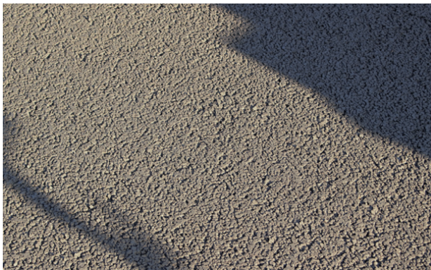
FIGURE 4. Detail of pervious concrete surface with D_{max} = 8 mm.
