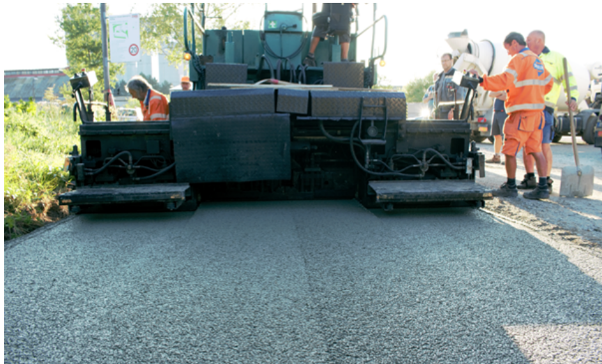
FIGURE 3. Laying down of pervious concrete.
