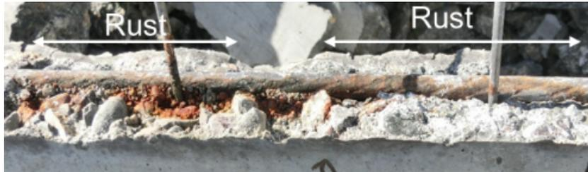
FIGURE 14. Observation of corrosion state of PC steel bar at the joint position of the concrete formwork during dismantling CP.
