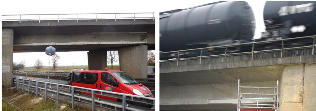
FIGURE 5. Strengthening of the railway bridge over the highway A70 under ongoing use on and under the structure.
