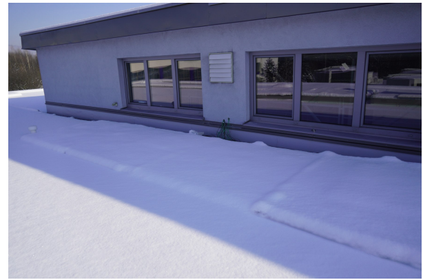
FIGURE 4. Roof covered with snow.
