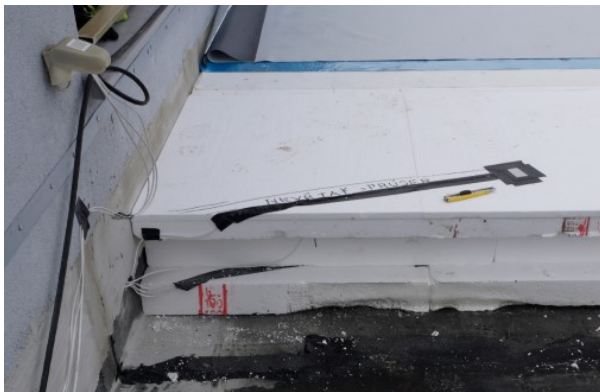
FIGURE 3. Incorporation the Sensirion SHT21 sensors during the reconstruction work.
