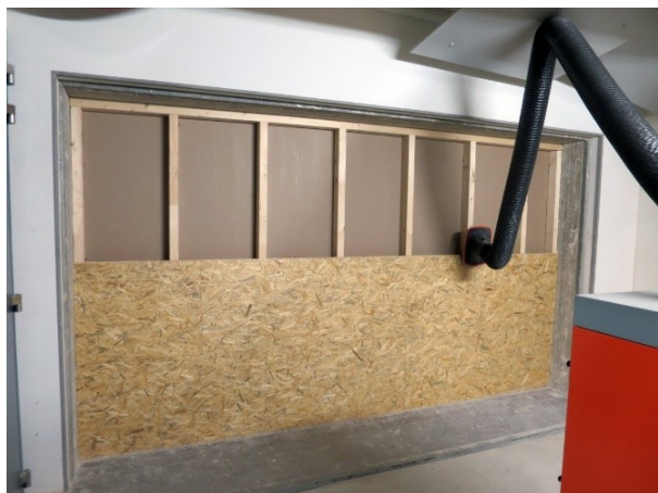
FIGURE 3. Filling the wall with crushed brick rubble (photo by K. Staněk).
