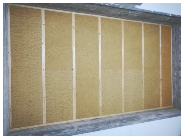
FIGURE 7. Wood fibre boards between I-joists STEICO wall.
