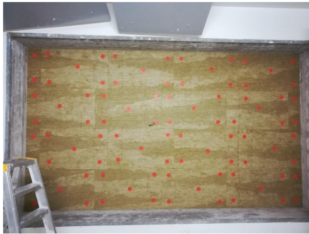
FIGURE 8. Mineral wool boards of ETICS fastened with anchors.
