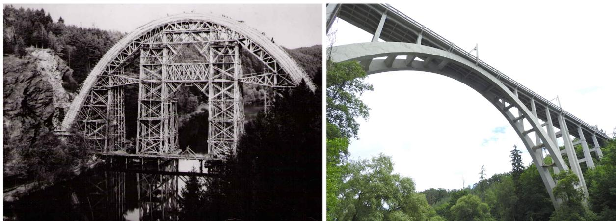
FIGURE 5. Arch road – railway bridge at Bechyně, 1928 (left – construction [6], right – at present).
