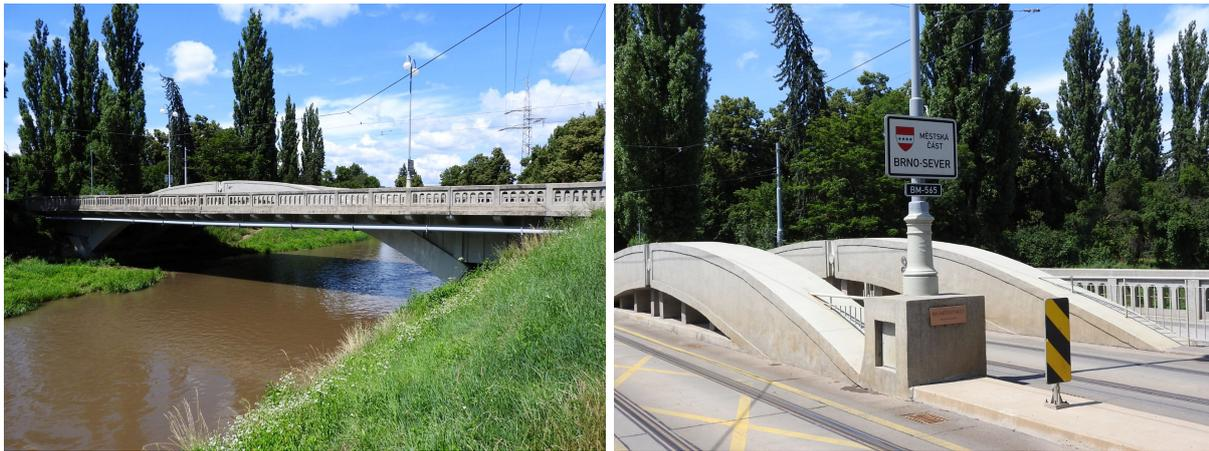
FIGURE 7. Three-hinge arch bridge at Brno – Husovice, 1928 (left – overall view, right – steel hinges).
