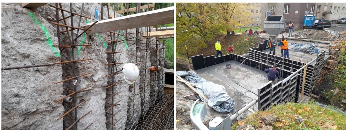
FIGURE 10. Ribbed UHPFRC layer around existing abutments and wing walls (left – preparation of the shape and reinforcement, right – casting the UHPFRC layer) – Meziboří at Litvínov.
