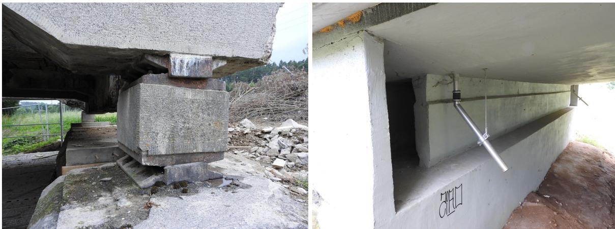
FIGURE 8. Pendulum supports (left – bow-string bridge at Bačkovice, 1929; right – end of the deck of the arch bridge at Přebyslav, 1940).
