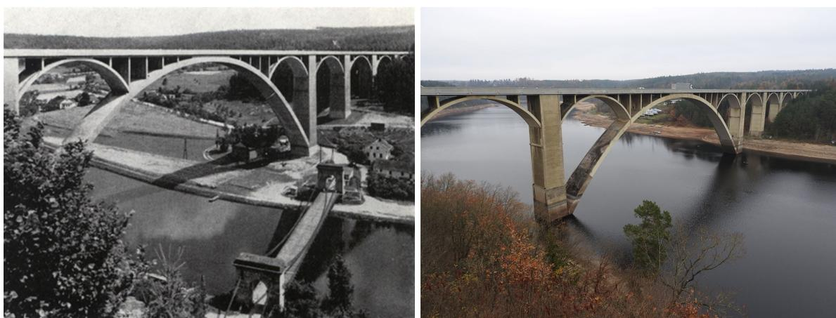
FIGURE 6. Arch bridge at Podolsko, 1939–1942 (left – during construction still with the former chain bridge [7], right – at present).
