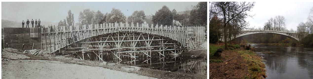
FIGURE 4. Vaulted bridge at Peřimov – Dolní Sytová, 1912 (left – during construction [5], right – at present).
