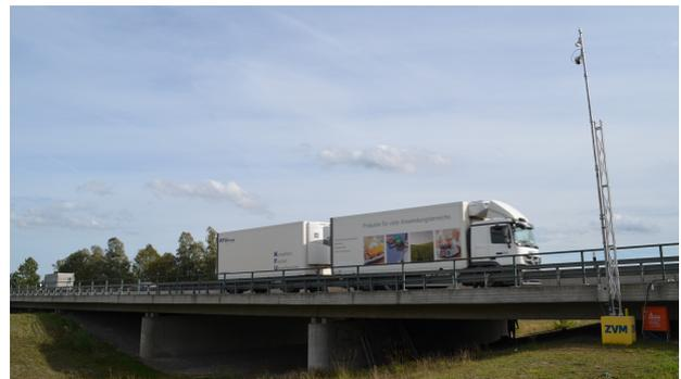
FIGURE 7. Traffic monitoring unit next to bridge.
