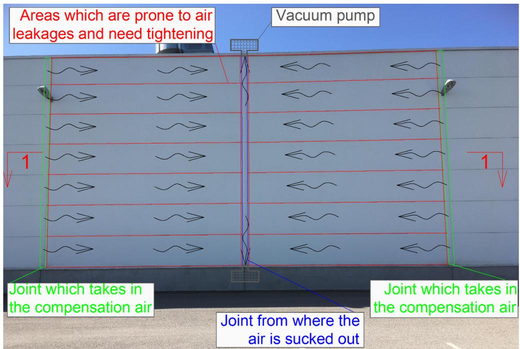
FIGURE 9. Scheme on facade for ventilated vertical joints and compensation air joints.
