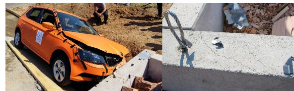
FIGURE 12. Deformation of drainage ditch with an integrated deformation zone after test No. 002.
