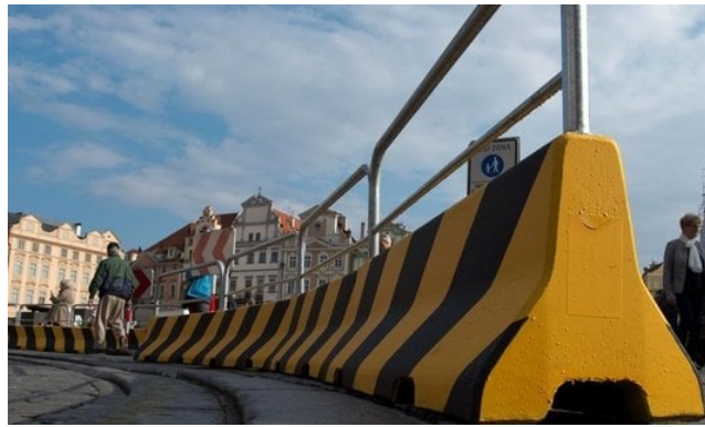
FIGURE 1. New Jersey crash barrier used in Prague [1].
