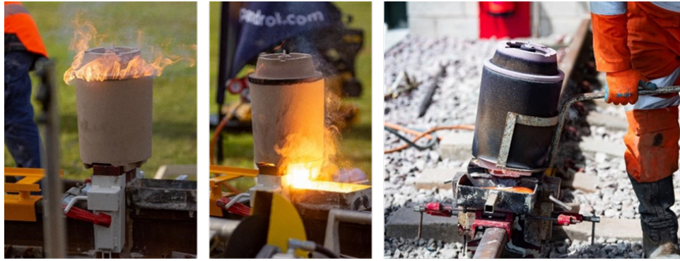
FIGURE 1. AT process of the PLA (Préchauffage limité) short pre-heating method using an automatic High Flow Preheating (HFP) unit and a one-shot crucible [13].
