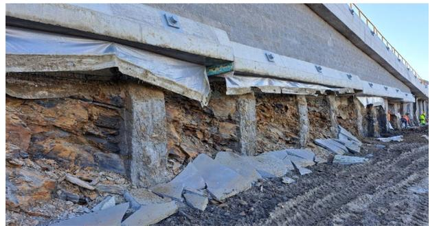
FIGURE 8. Exposed panels with visible beams and anchors.
