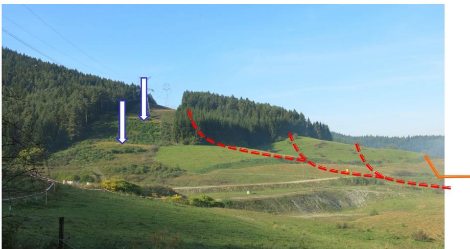
FIGURE 3. Distinct morphological blocks of rocks under the power line (blue arrows) and a diagram of blocks with shear surfaces (red lines).
