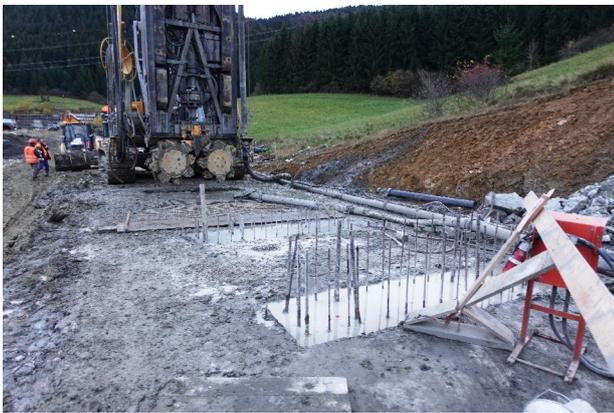
FIGURE 7. Excavation for the diaphragm wall panels with width of 2.8m.
