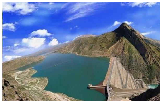
FIGURE 1. General overview of the dam.
