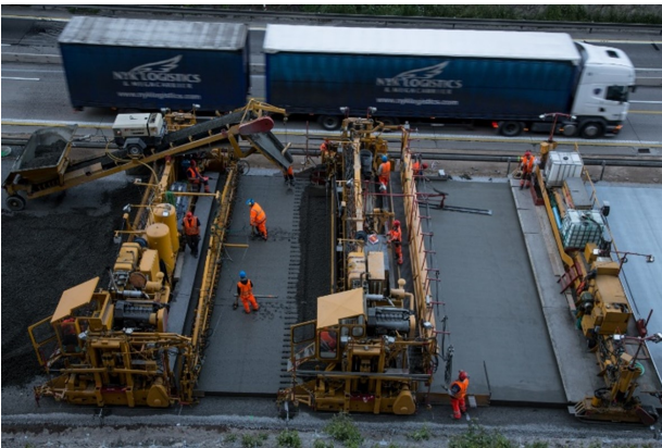
FIGURE 6. Finisher set for two-layer cement concrete pavement, construction D1 (STRABAG).
