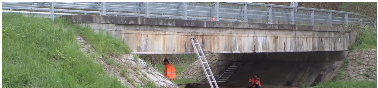
FIGURE 3. View of bridge.
