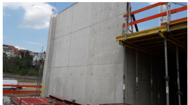
FIGURE 10. A 8 m high wall made from SCC-5 % MK mixture.
