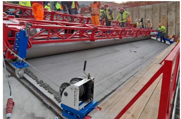
FIGURE 5. Finalisation of the surface.
