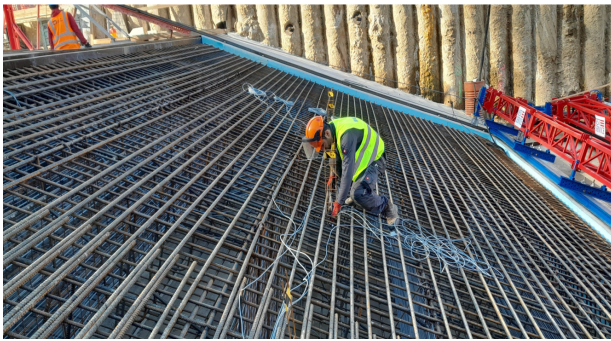
FIGURE 6. Installation of strain gauges at the construction site.
