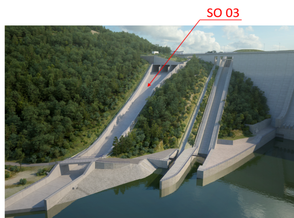
FIGURE 1. Visualisation of the open part of the chute spillway (SO 03 on the left) [5].
