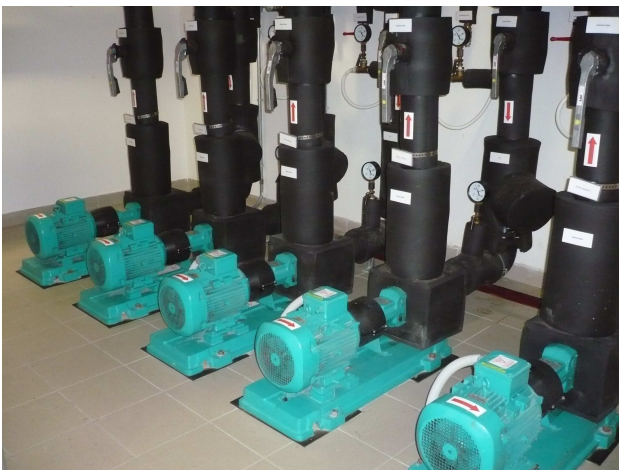
Fig. 5. Circulation Pump in the Primary Circuit, 5 units
