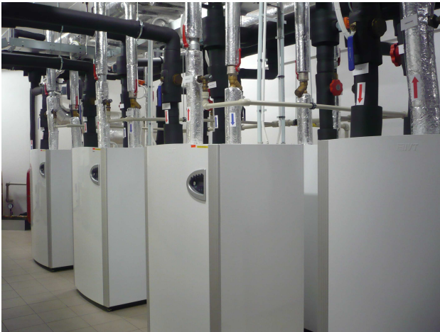
Fig. 4. Heat Pumps, 10 units
