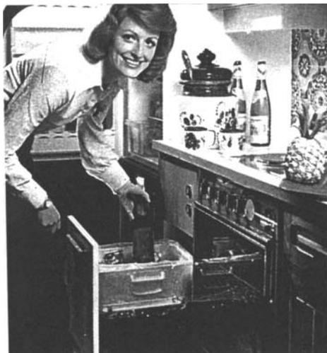
Fig. 1: The Lescha-Mollpack waste baling press integrated into kitchen furniture
