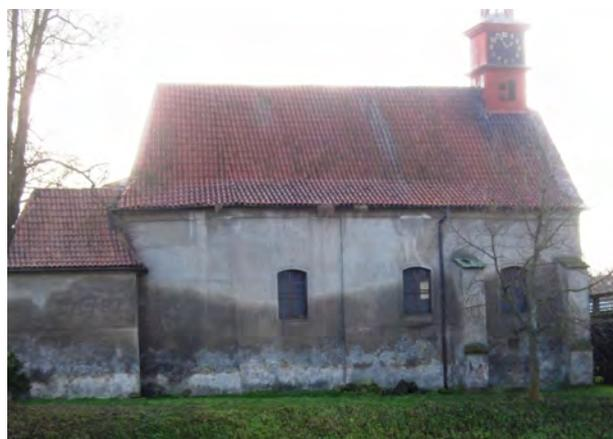
FIGURE 1. Long-term effect of rising moisture (unmaintained historic building) — Church of St. Catherine (built in 1315, modified in 19th century), Havlickuv Brod, CZ.
