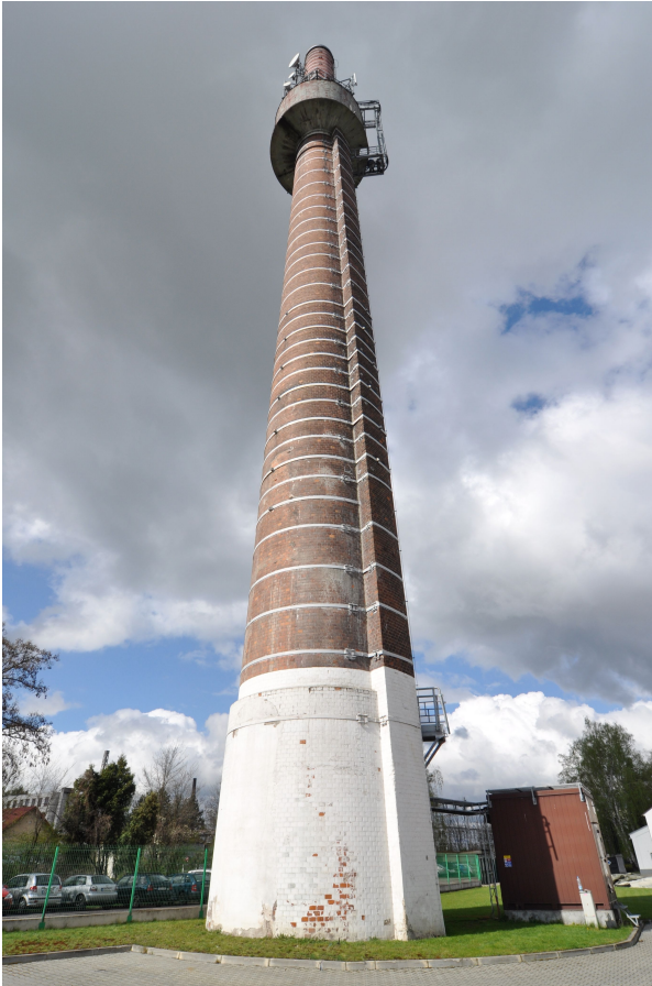
FIGURE 9. An example of a brick piping shaft, 2014.
