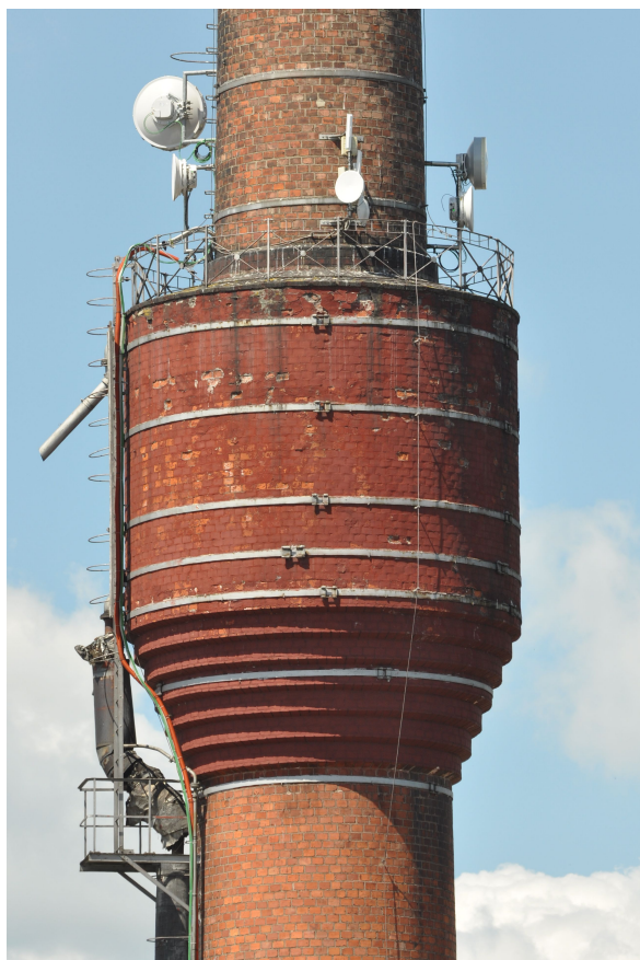
FIGURE 7. The only known brickwork reservoir on the territory of the Czech Republic – the flax and cotton mill in Sudkov (built in 1908), 2015.
