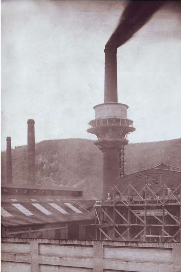
FIGURE 5. The construction of a reinforced concrete reservoir built onto a functioning chimney at the screw factory in Libčice, 1921 [24].
