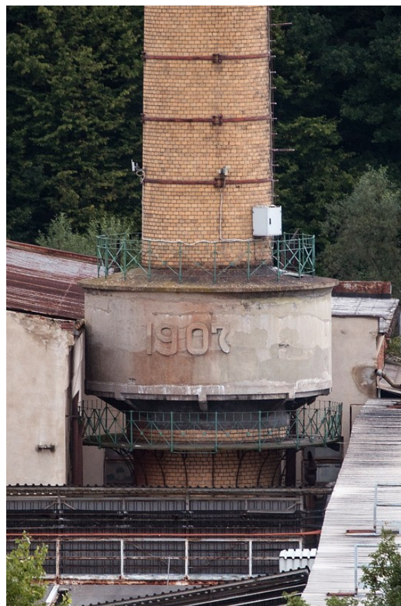
FIGURE 8. The first reinforced concrete chimney reservoir – the paper mill in Olšany (built in 1907, demolished in 2016), 2013.
