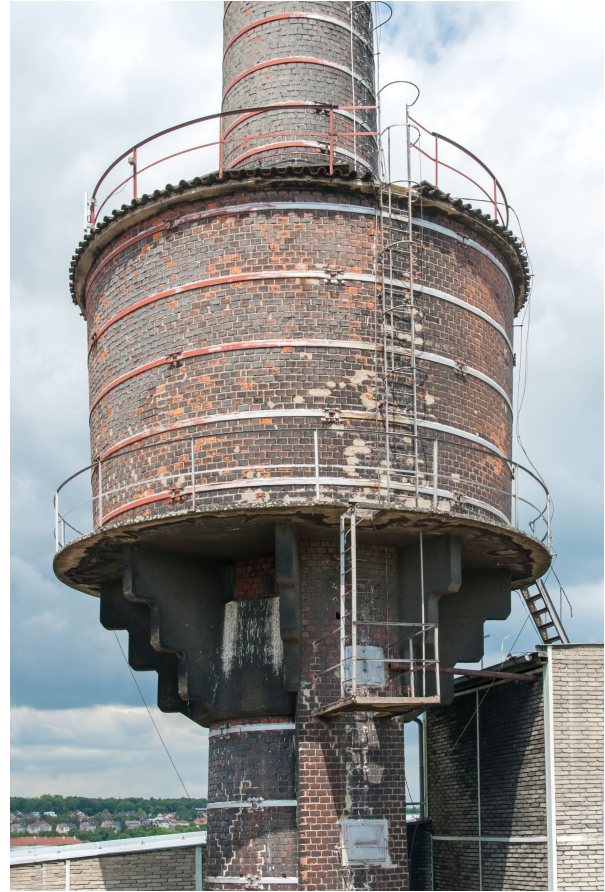
FIGURE 6. A reinforced concrete reservoir built onto a chimney in Slaný, 2013.
