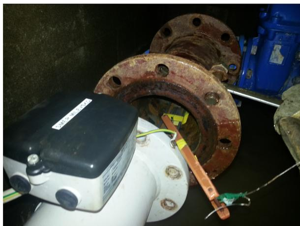
FIGURE 3. Removal of the plates after the required exposure time
