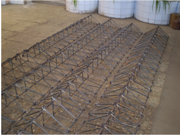
FIGURE 2. The look of spatial reinforcement frames of sandwich reinforced concrete-foamed concrete floor slabs after manufacturing.
