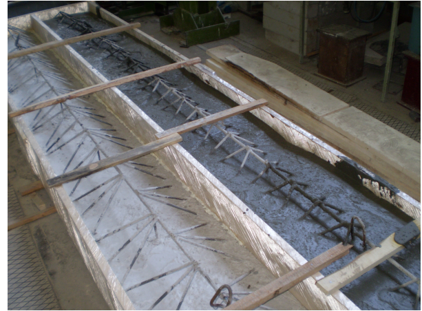
FIGURE 4. The look of sandwich reinforced concrete-foamed concrete floor slabs during concrete casting by foamed concrete or foamed concrete with fibre polypropylene.
