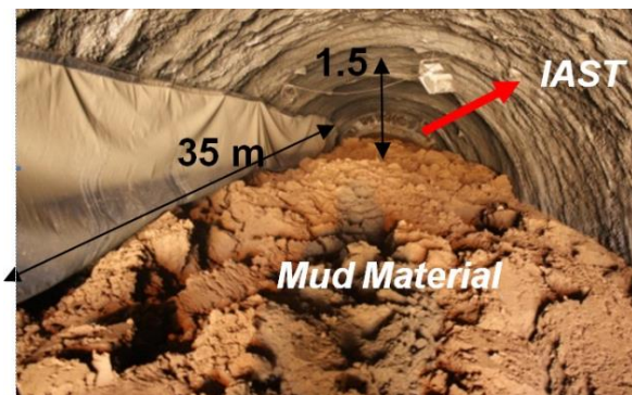
FIGURE 11. The mud flow running into the tunnel.
