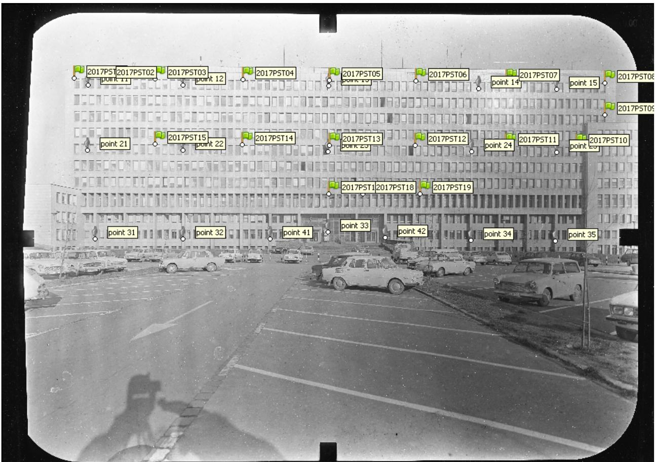
FIGURE 2. Distribution of ground control points on the main facade of the “Post Office Palace”.
