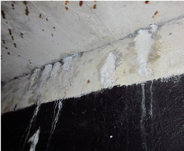
FIGURE 10. Surface efflorescence in the interior (bunker R-S-74).
