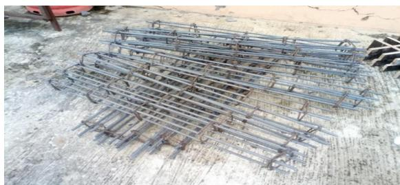
FIGURE 3. Y10 Beam Reinforcement.
