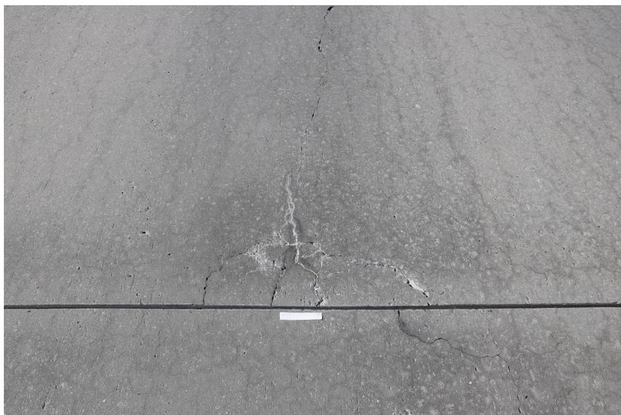
FIGURE 11. Accelerated damage of concrete highway (D5 9-20 km) determined by cracks induced by the shrinkage.
