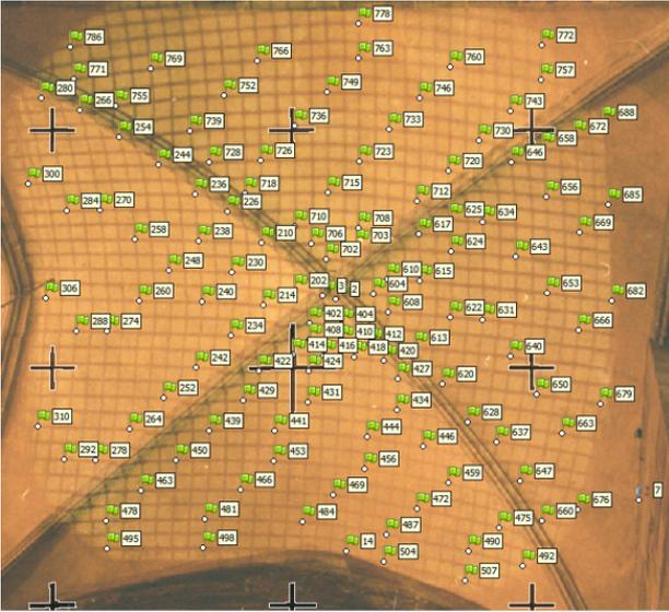
FIGURE 10. Distribution of check points on the vault.
