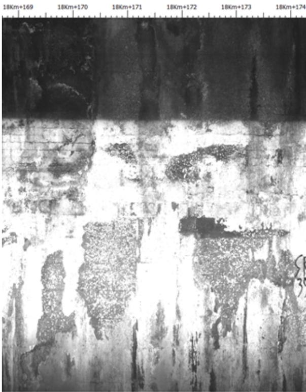
FIGURE 11. Detachment of concrete cover and exposure of the rebars (yellow area).
