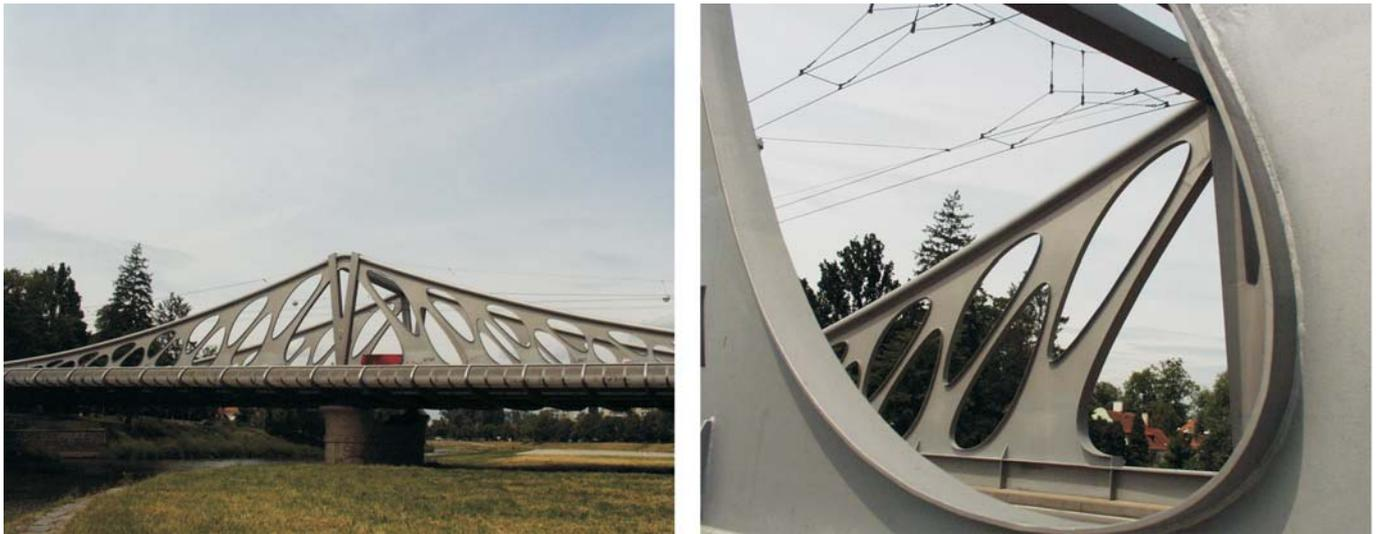
Fig. 10: Long Bridge in České Budějovice. Built 1999 by Roman Koucký and Tomáš Rotter. The structure of the bridge (left). The rubber-like deformed openings of the side beams (right). (Authors of figures: Lenka Popelová and the database of the VCPD, CTU in Prague.)
