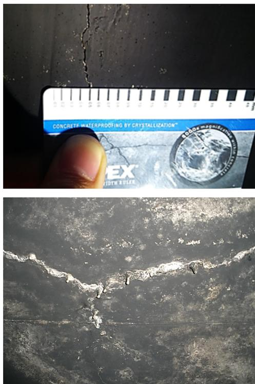
FIGURE 8. Flexural cracks with a width of 0.4–0.5 mm found on the bottom face of the RC slab above the underground floor (top) with observed leakage of fire-extinguishing water (bottom).
