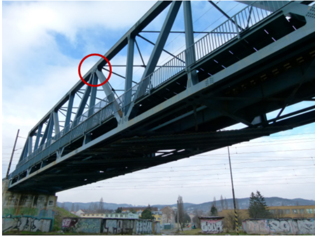
FIGURE 7. Exact point of the bridge structure monitored by IBIS-S radar.
