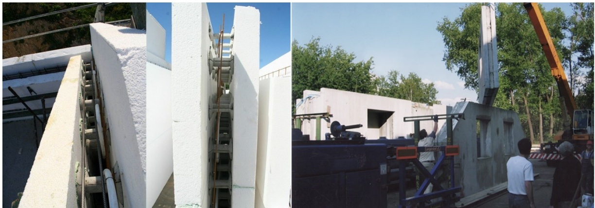
FIGURE 3. Left and centre – ISOMAX thermal barrier (TB) perimeter panel made of lost-foam expanded polystyrene formwork, on the right – panels comprehensively manufactured in the panel factory [7].
